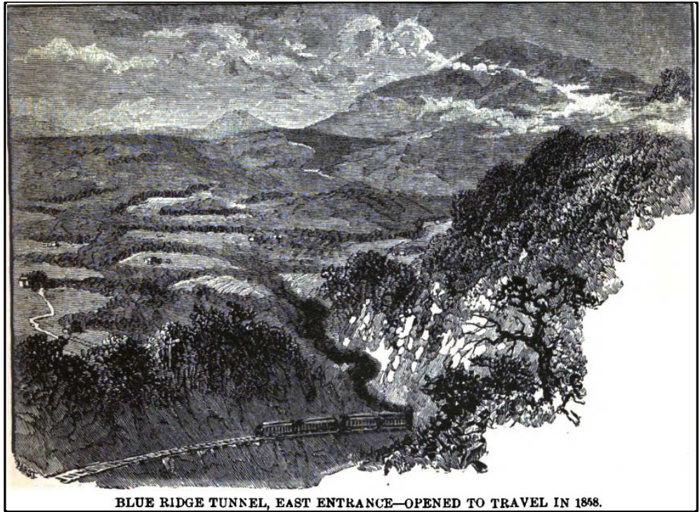
BLUE RIDGE TUNNEL, EAST ENTRANCE—OPENED TO TRAVEL IN 1858.
