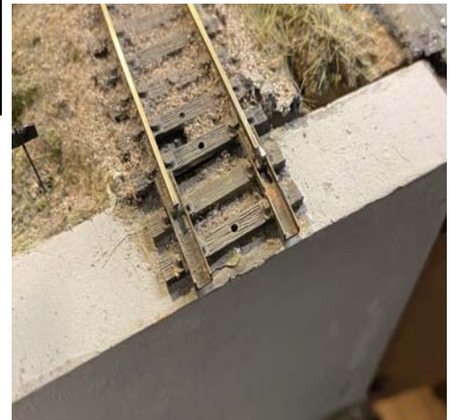
1/8" brass U channel solder to the base of the rails, helps guide the adjacent bridge track into alignment.
